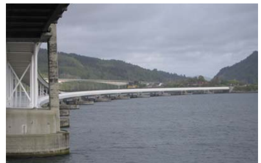
Nord Hordland Bridge
